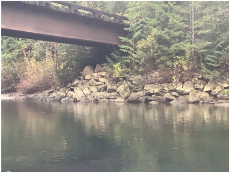
Right Bank Abutment when facing downstream
