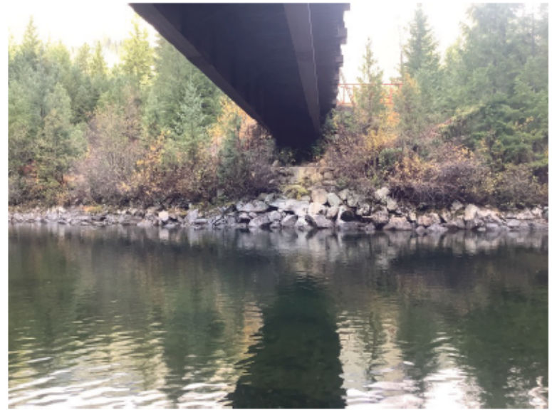
Left Bank Abutment when facing downstream
